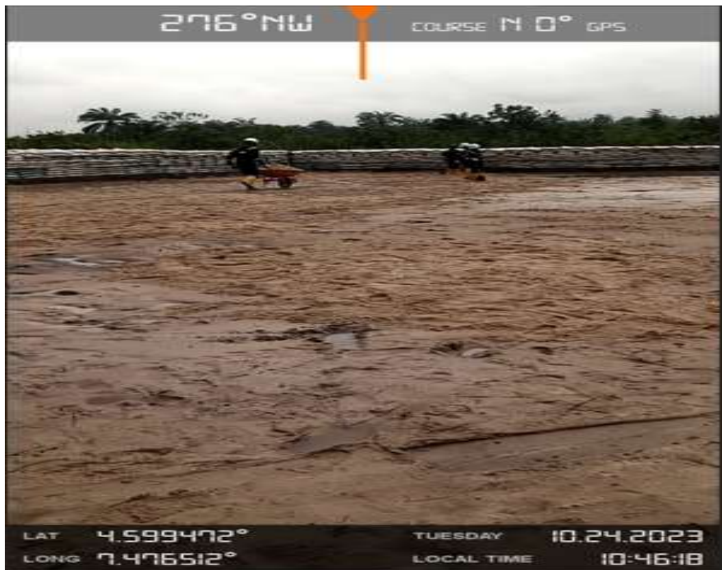
Plate 1: Sand filling of Biocell floor for Slopping Ongoing
