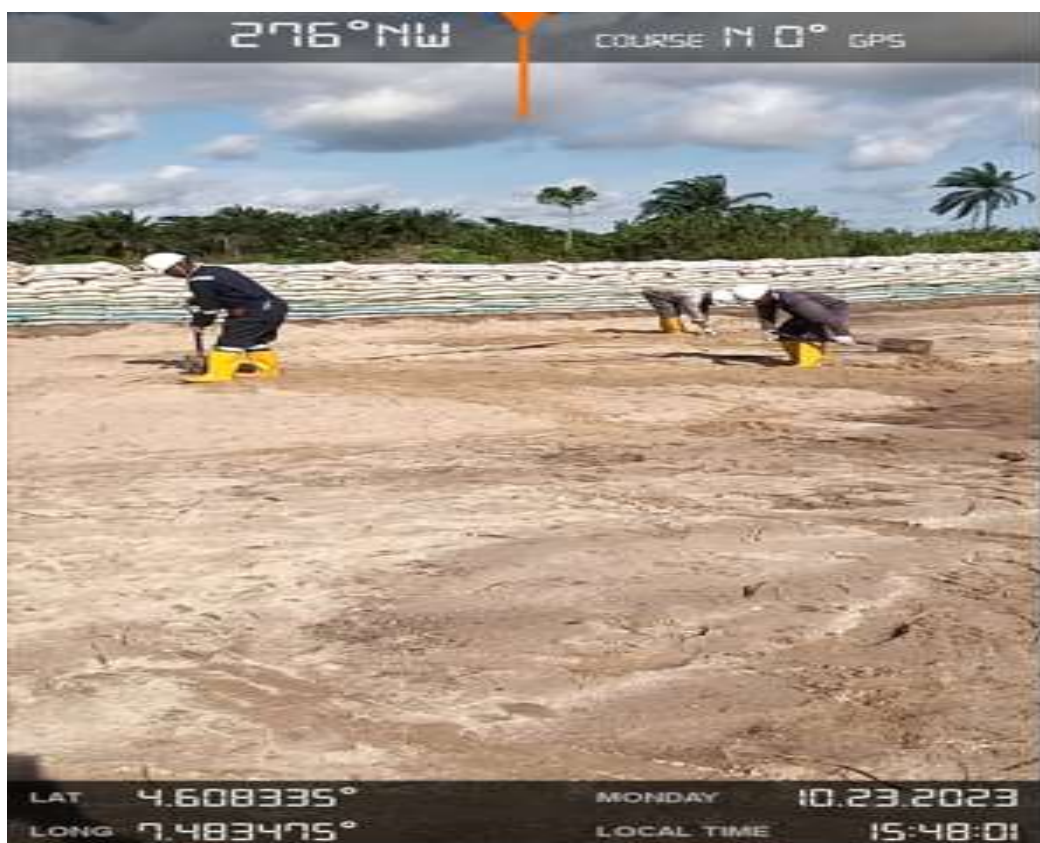
Plate 2: Levelling and Slopping of Biocell Floor
