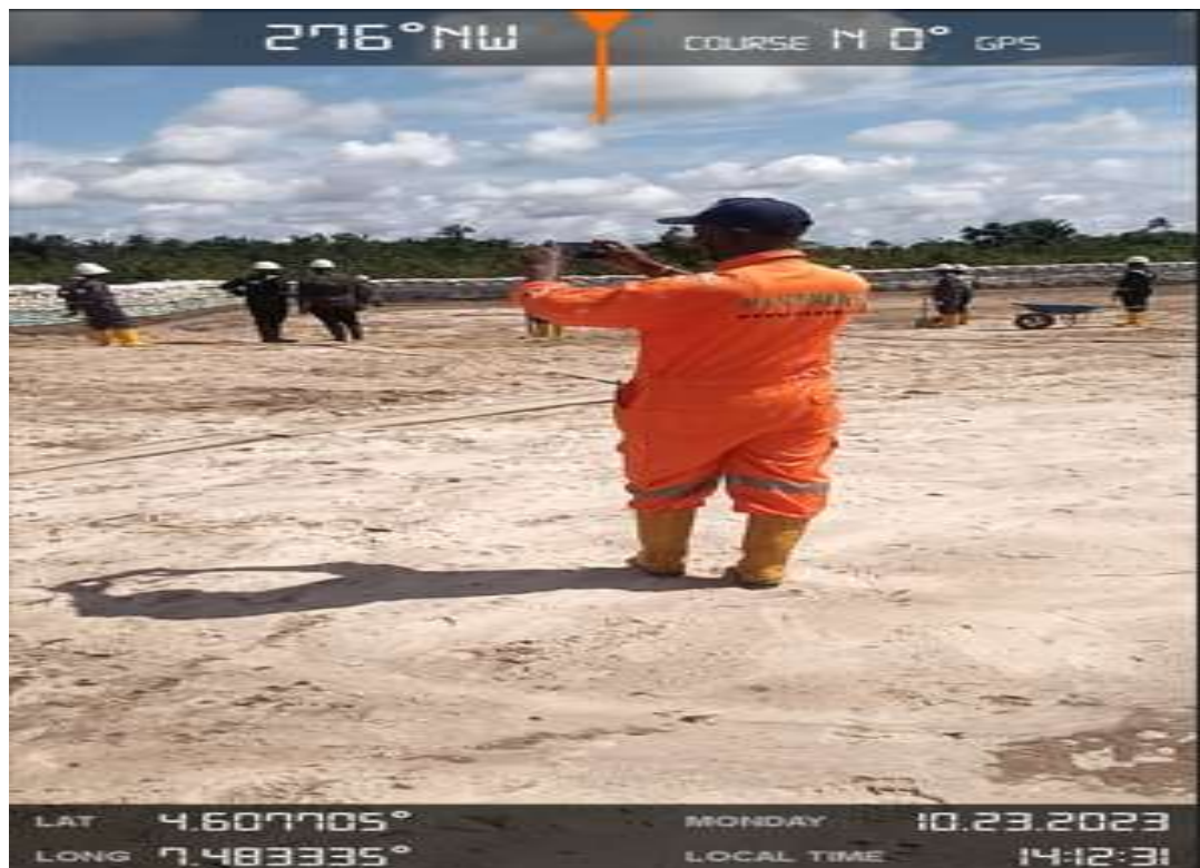
Plate 4: Hyprep Site Supervisor Inspecting ongoing Activities
