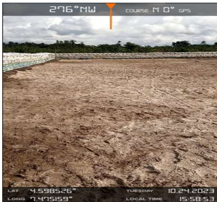
Plate 8: An Overview of Completed Biocell Laying of Sandbags
